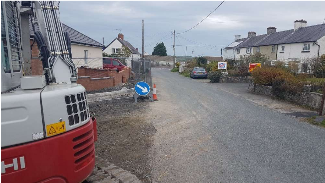
View from the access looking north.
