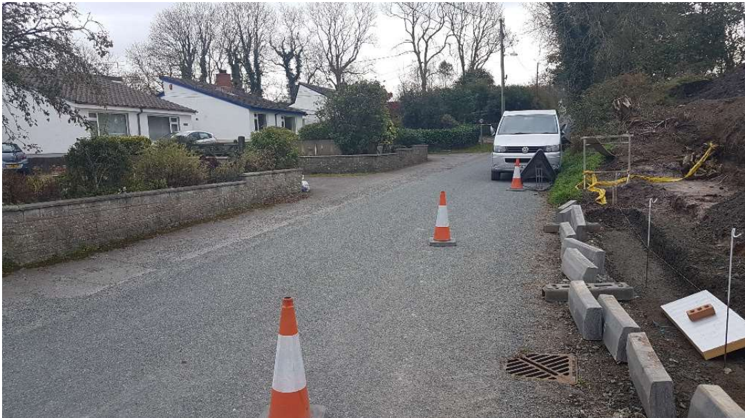
View from the access looking south.
