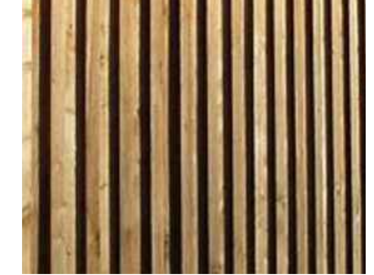
WALLS VERTICAL TIMBER BOARDING
